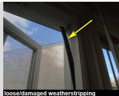
loose/damaged weatherstripping
