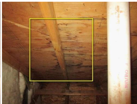
stains from flashing leak
