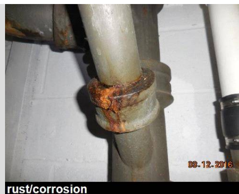
rust/corrosion
