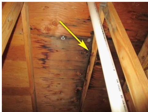
stain from flashing leak
